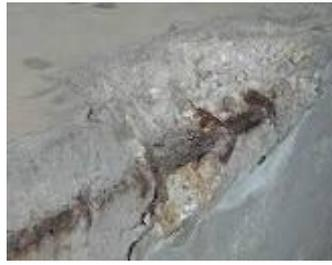
The corrosion is an electrochemical nature process. And the presence of an electrolyte requires like all the electrochemical processes to be able to produce himself. In concrete case the electrolyte is the solution present in his capillary pores which is substantially a sodium and potassium hydroxide solution with a pH included between 13 and 14.
